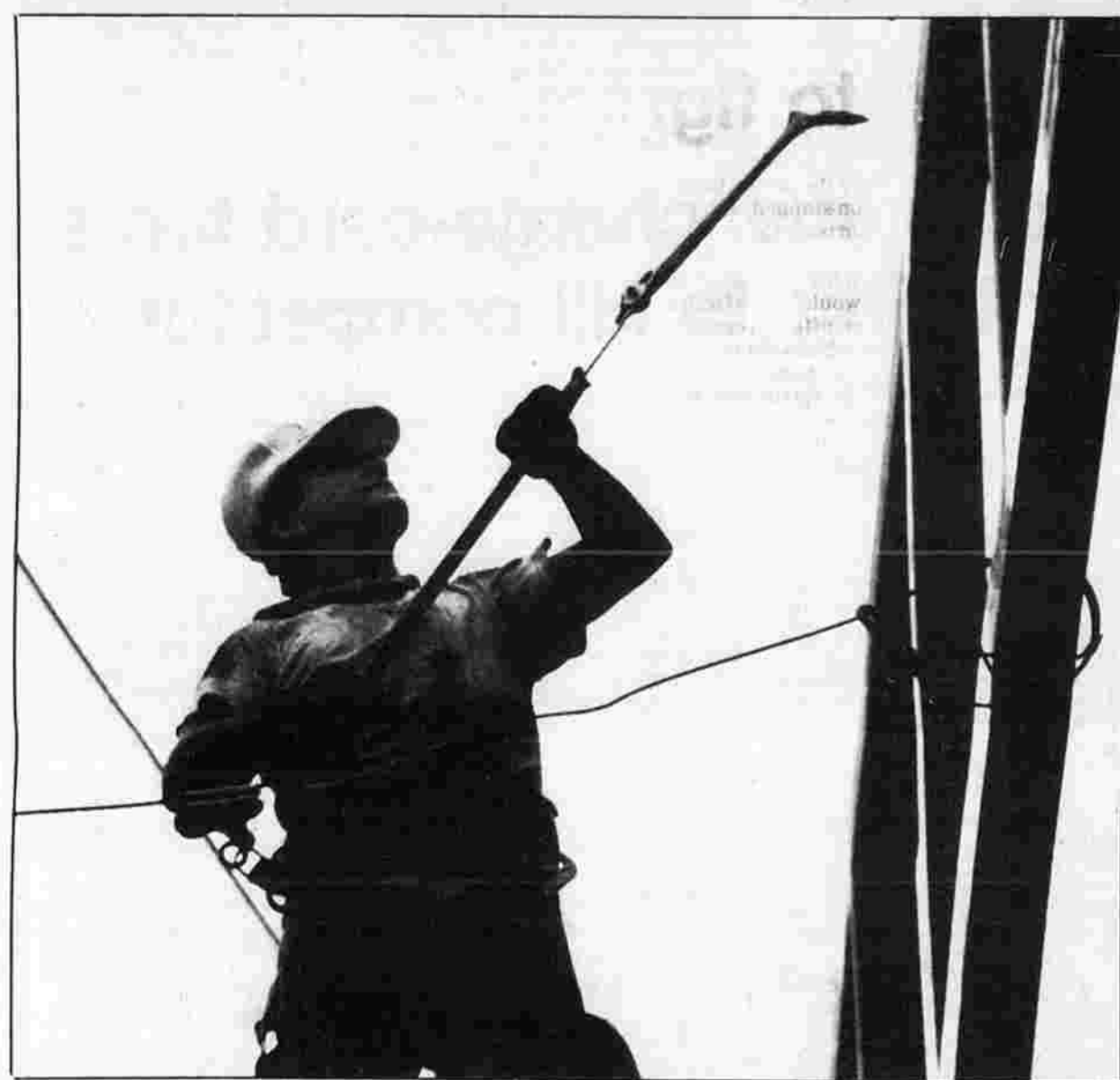
PREPARING TO PAINT — John Obiden of Wolcott, a painter, scrapes an area outside the mall before painting it Wednesday. The $70 million mall is scheduled to open next spring and will include its own police substation.
