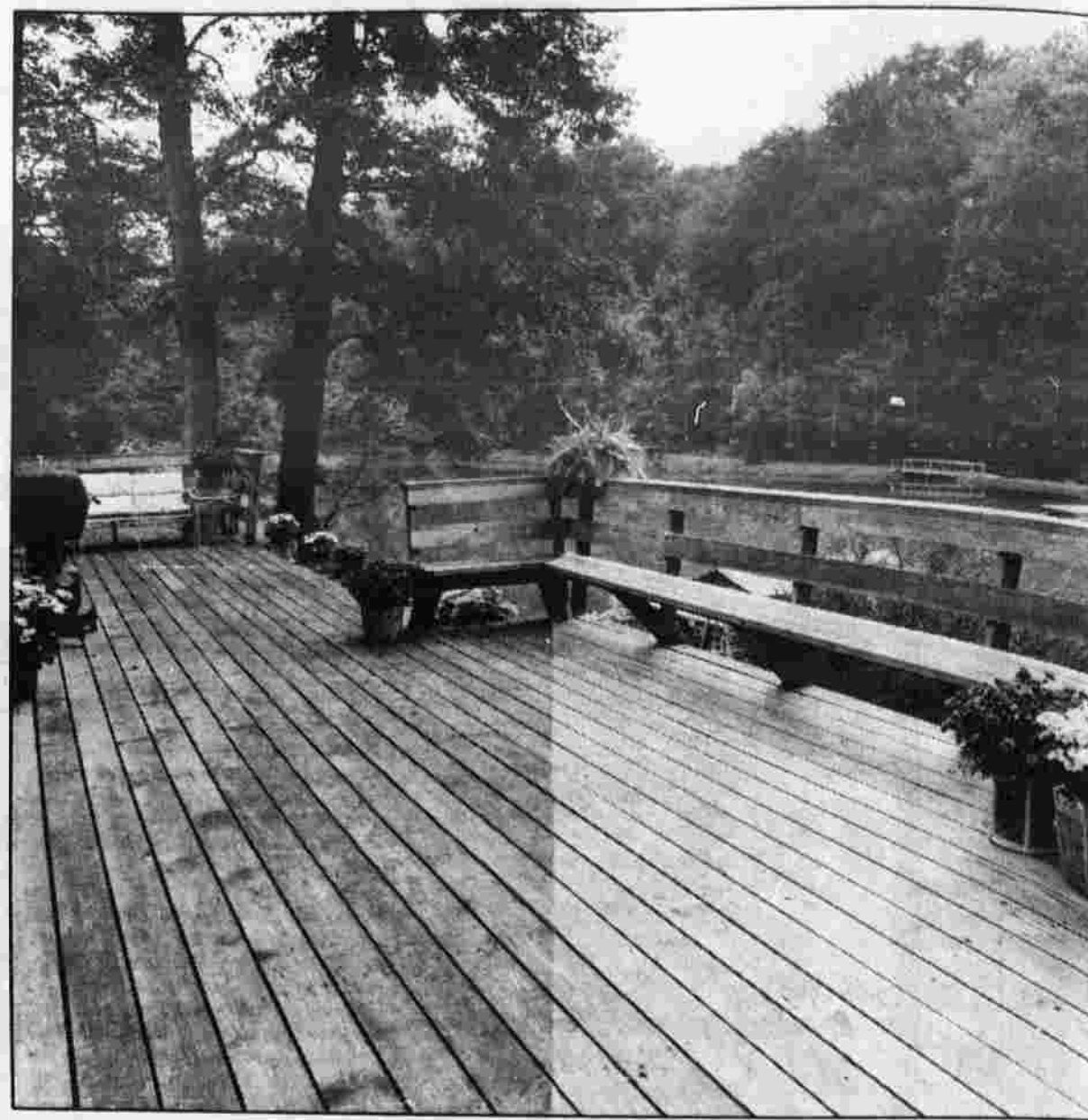
RESTORING A DECK — Restoring a deck is easier with the use of a water repellent. The right side of the deck has been restored, while the left side has been beaten from eight years of rain, snow, sun and wind.
